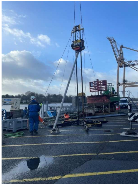
Figure 3-5 Core barrel being lifted in place by crane
